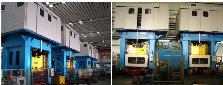
Fig. 6. Noise level of individual machines was reduced by sound insulated enclosures
