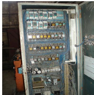
**Fig. 7** Cabinet with contactor equipment
