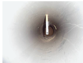
Fig. 3. The inner surface of primary air duct with transmitters
