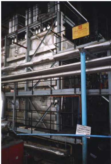
Fig. 5. Boiler with power 30 MW
