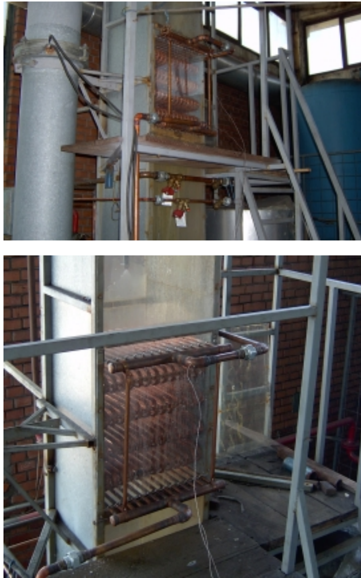
Fig 4. Photos of experimental installation
