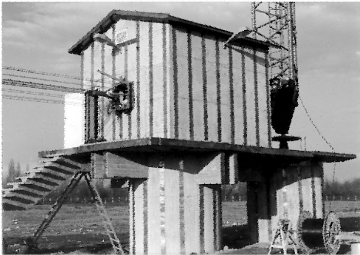
Picture 2. A detail of elevated antenna base.
