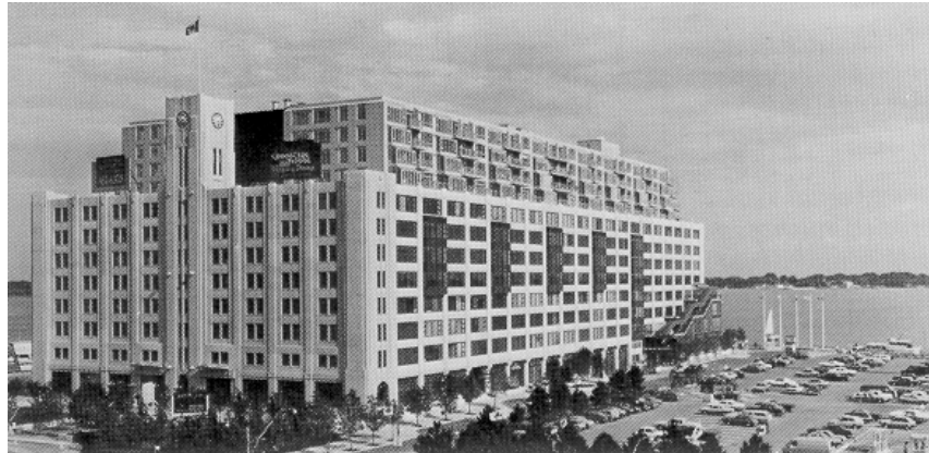
Fig. 2. Queen's Quay Terminal, Toronto North-west elevation after renovation
