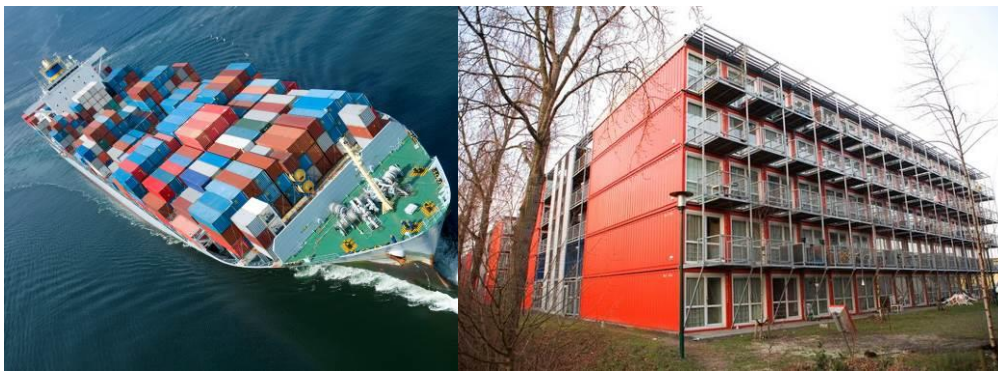
Fig. 7 Container ship and Keetwonen recycled container student housing in Netherland
