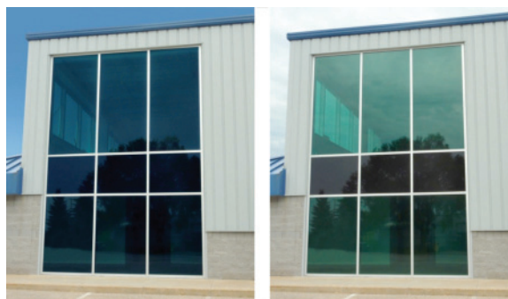
Fig. 4. Sunlight responsive thermochromic glass: (a) windows are tinted by direct sunlight; (b) windows are clearer as they are only exposed to indirect sunlight
