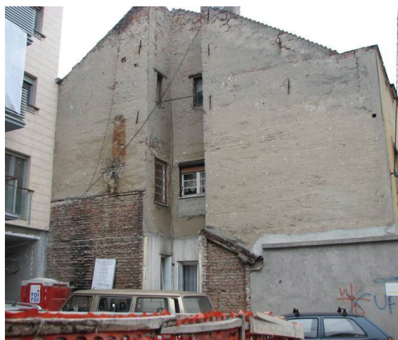
Fig. 2 Side (gable) wall of the old house
