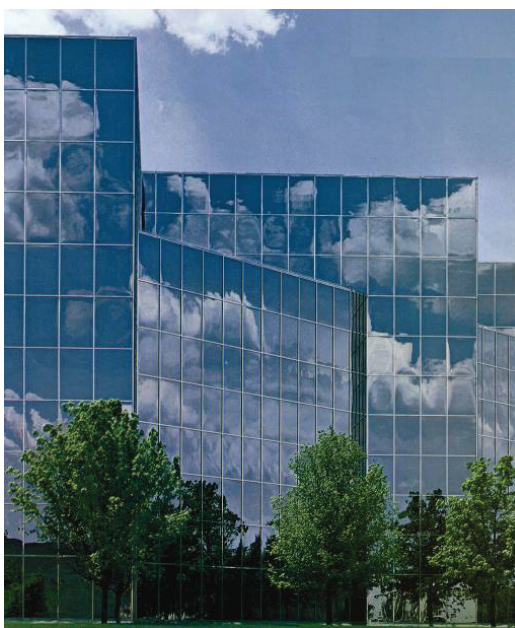
Fig. 2. Office building facade clad in "EC" glazing.
