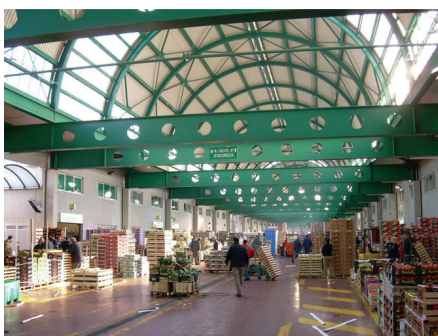
Fig. 8. Central corridor interior view
