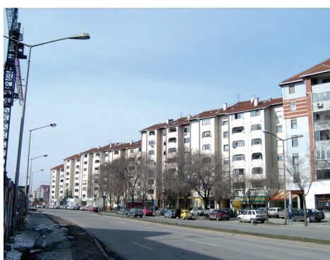
Fig. 12. Building block F4
