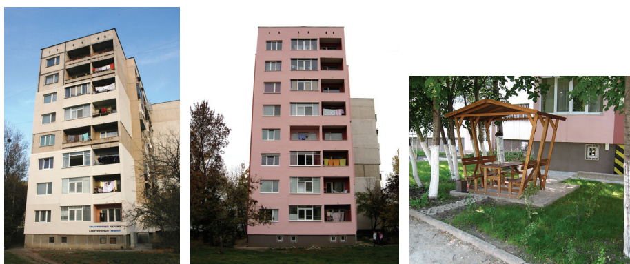
Fig. 5-7. Façade before and after refurbishment and surrounding, after [28]
