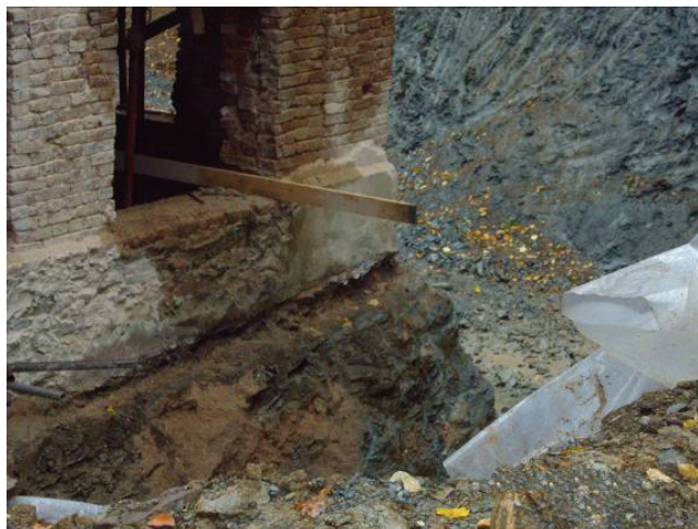
Fig. 6. Wide excavation of the structure prepared for the execution of the remediation cut at the base of the wall construction
