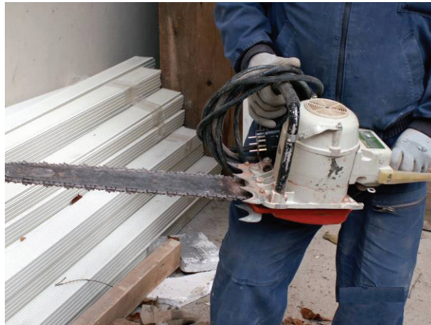
Fig. 14. Auxiliary manual cutting hand-held saws for a possible correction of irregularities of the joint cut or widening of an already existing joint in the wall construction
