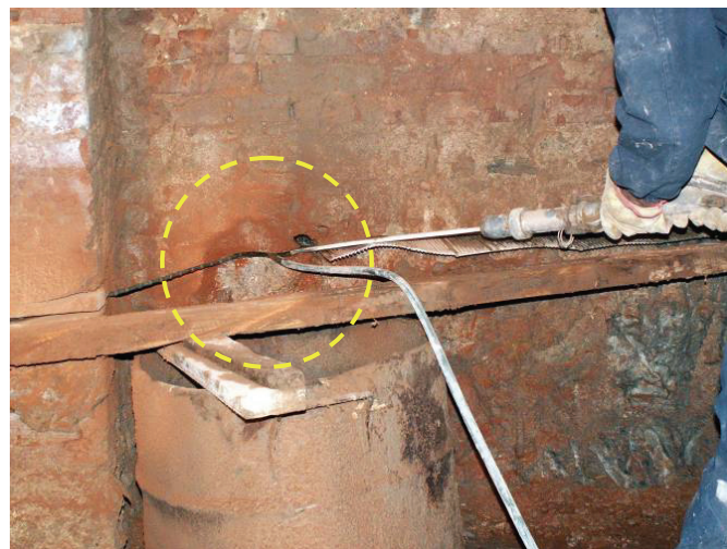
Fig. 9. Blowing and wetting of the joint during the masonry cutting process
