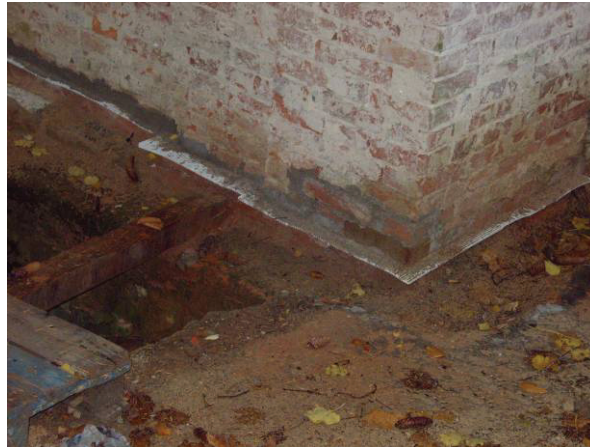
Fig. 16. Total waterproofing barrier constructed in the corner part of the wall structure
