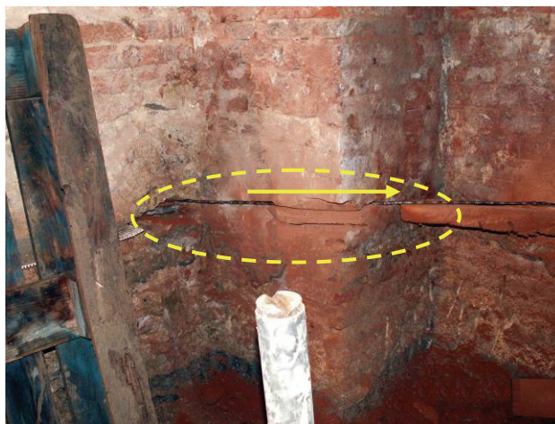
Fig. 10. View of the wall section being cut
