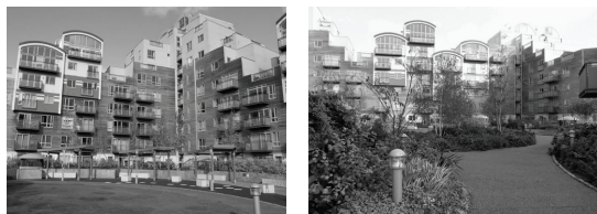
Fig. 7 Maurer Court, Greenwich Millenium Village, UK, E. Tovatt, EPR Arch.; 2003
