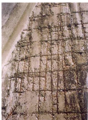
Fig. 9 Cooling tower mantle
