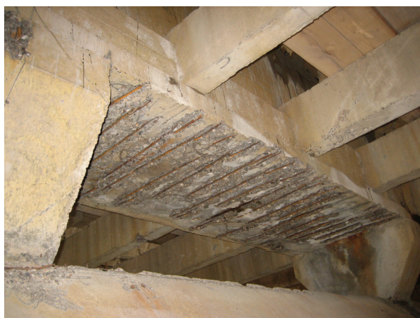
Fig. 10 Beam for sprinkler installation
