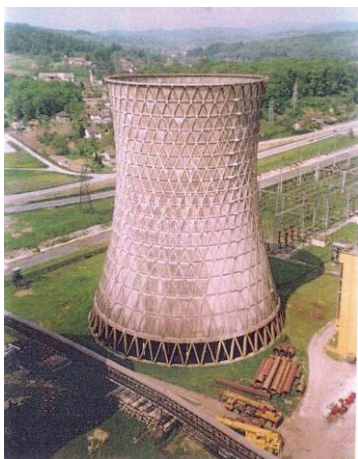
Fig. 11 Cooling tower, Thermoelectric Power Plant in Tuzla
