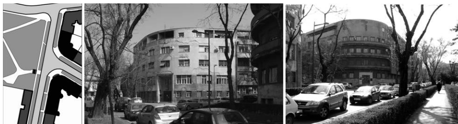
Fig. 7 Corner built-in buildings across the park
