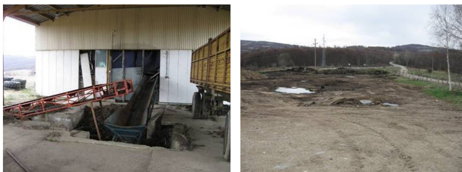
Fig. 5 Peat processing plant (left) and peat store area (right) next to the previously factory mentioned
