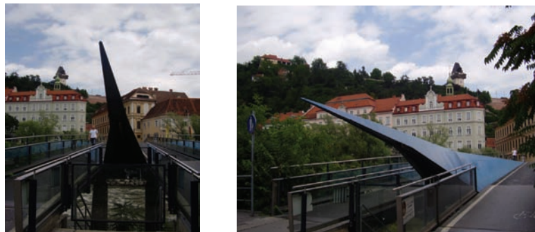
Fig. 7 Mursteg- pedestrian Bridge Photo made by author
