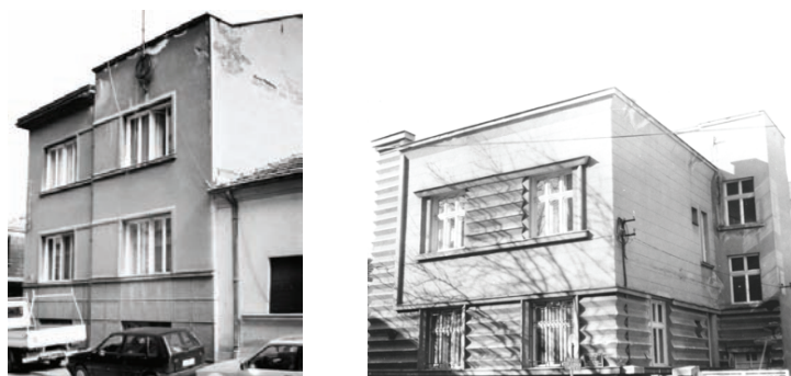
Fig. 19 Various forms of putting frames around the window apertures
