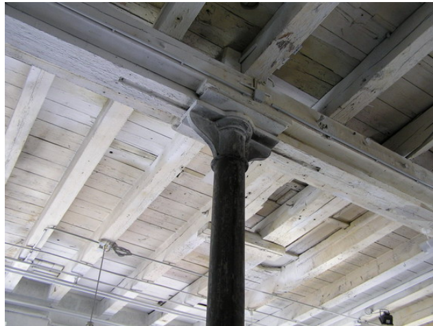
Fig. 2. Cast iron column supporting timber floor
