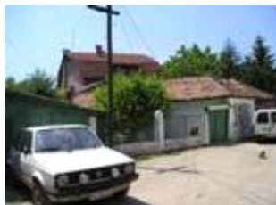
Fig. 8. Absence of height alignment
