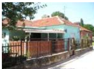
Fig. 5. Structure bordering the street
