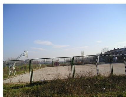
Fig. 24. Enclosed sport courts
