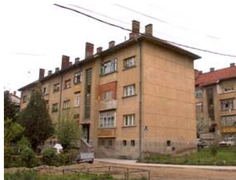
Fig. 6. Appearance of the building prior to heightening viewed from the northwest side
