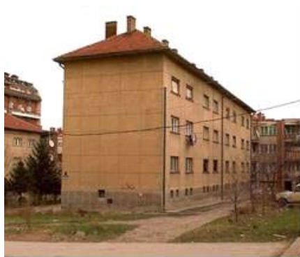
Fig. 5. Appearance of the building prior to heightening viewed from the southwest side
