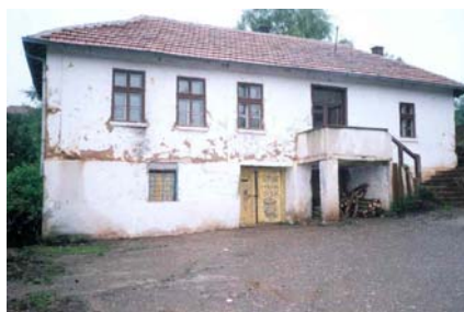
Fig. 5. Characteristic façade of the old type school building, 1946, Leskovik village
