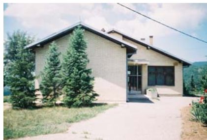
Fig. 6. New school building façade of 1972, Knez selo
