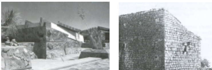
Fig. 29. Similarities in application of stone at Wright and the House of Pastrovici
