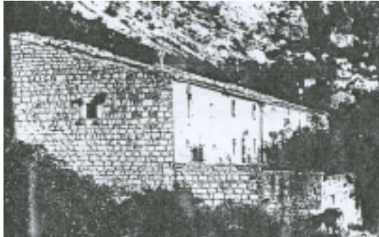
Fig. 10. The example of the lean-to roof
